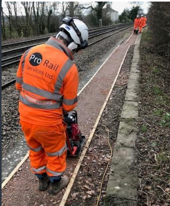
BLACKBROOK SUBSTATION, DORKING, SURREY
